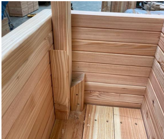
Planter showing corner post sleeves to hold the posts GRP/Fibreglass planters have a similar support sleeve
